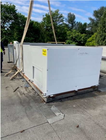
New RTU 1&2 (Maple Creek): New RTUs installed at Maple Creek Middle School.
