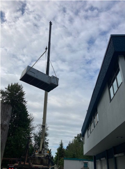
New RTU 1&2 (Maple Creek): New RTUs installed at Maple Creek Middle School.
