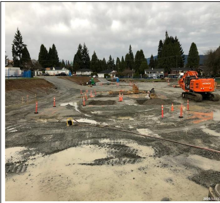
They have completed ESC (Erosion and Sediment Control) work, site fencing is in place, Como Lake storage shed has been demolished and removed from the site and much of the bulk excavation, footings formwork and pouring of foundation footings has taken place or is underway.
