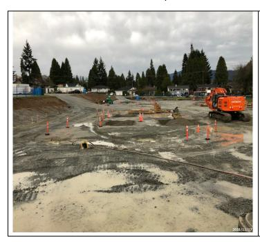
They have completed ESC (Erosion and Sediment Control) work, site fencing is in place, Como Lake storage shed has been demolished and removed from the site and much of the bulk excavation, footings formwork and pouring of foundation footings has taken place or is underway.
