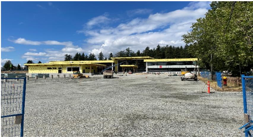
Currently compaction work is ongoing on the parking lot in preparation for asphalt scheduled to be late in the summer. The image shows the bases of columns for what will be a covered walkway with parking spots for electric cars and chargers.
